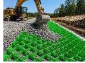
AGGREGATE INFILL FOR LOAD SUPPORT
