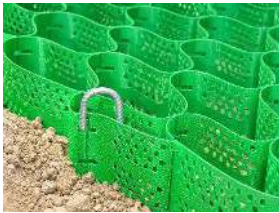
FIELD INSTALLATION OF MECHANICAL ANCHORS
