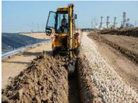
PREPARED CONSTRUCTION SUBGRADE AND ANCHOR TRENCH
