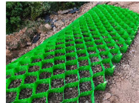
FIG 02 - EXPANSION GEOMETRY AND PINNING
