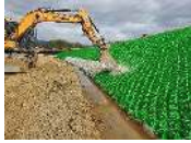
VEGETATED SLOPE TOPSOIL INFILL
