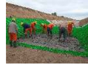
CONCRETE CHANNEL LINING INFILL
